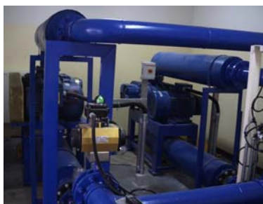
Enclosures ,Silencer, In line filter ,Control valve, All installed in the blower room
