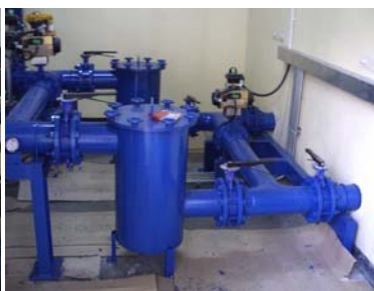
Enclosures ,Silencer, In line filter ,Control valve, All installed in the blower room
