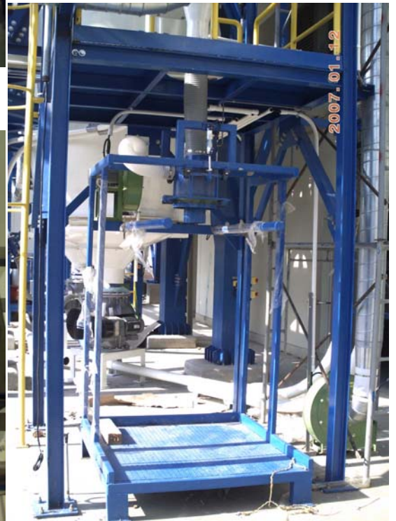
Bulk Bag Loading Station for paper pulp chip (raw material for dynamite bomb)
