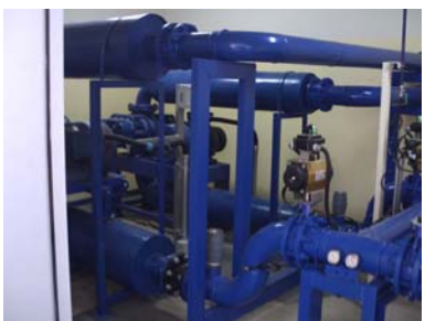
Enclosures ,Silencer, In line filter ,Control valve, All installed in the blower room
