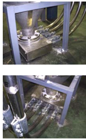
Collecting hopper & Outlet Box,SUS304
