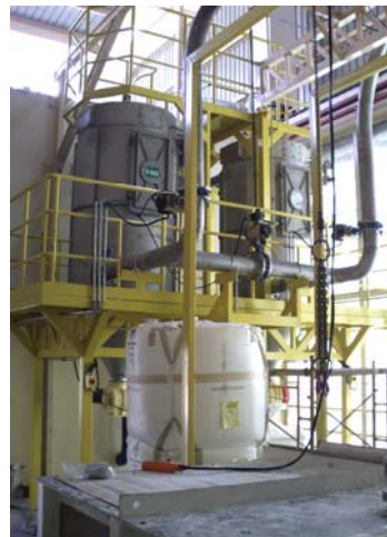
Dumping Hopper ,Ejector , Flexible hose, and Quick coupling from Extruder
