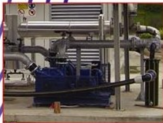
Multi-stage Centrifugal Blower
