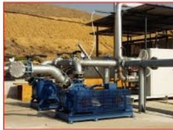
Multi-stage Centrifugal Blower
